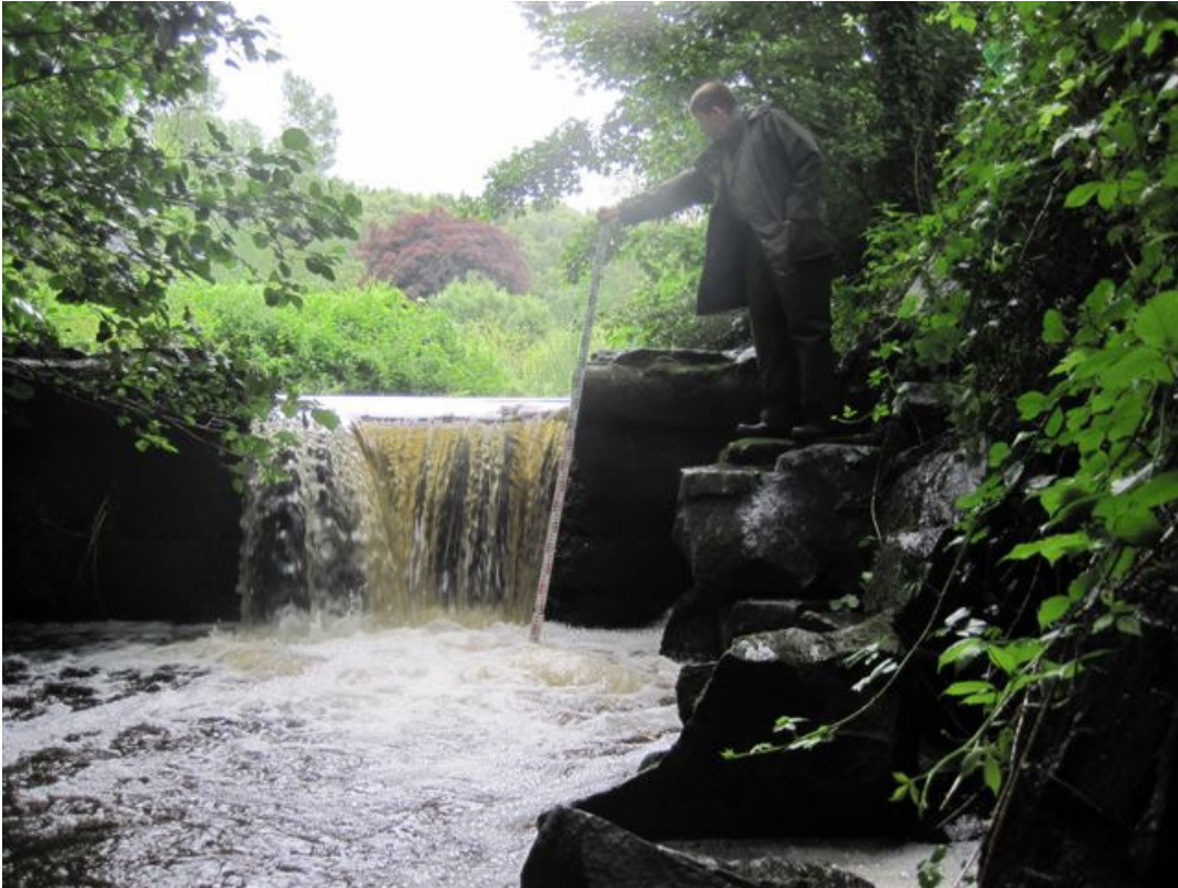
Figure 28. Dam across the Ballyduff Stream a close to Arklow. Original purpose of this dam believed to be the creation of a fish pond. Structure represents an impassable barrier to all fish passage, with excellent salmon spawning/nursery habitat upstream.
