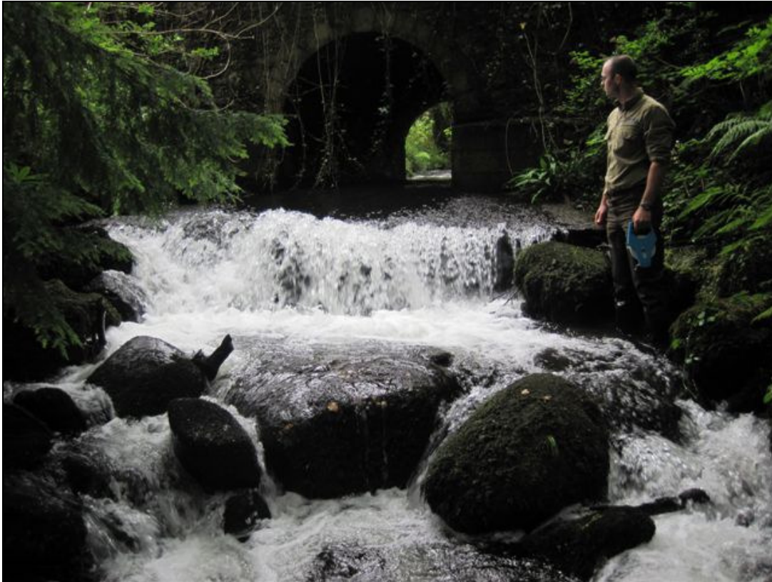
Figure 13. Photo of Ballyhad Bridge apron (Avonmore system: showing the perching, laminar flow and high velocities associated with this structure). Excellent salmon nursery habitat upstream. Site would also benefit from a mammal pass on this very busy/fast stretch of road.
