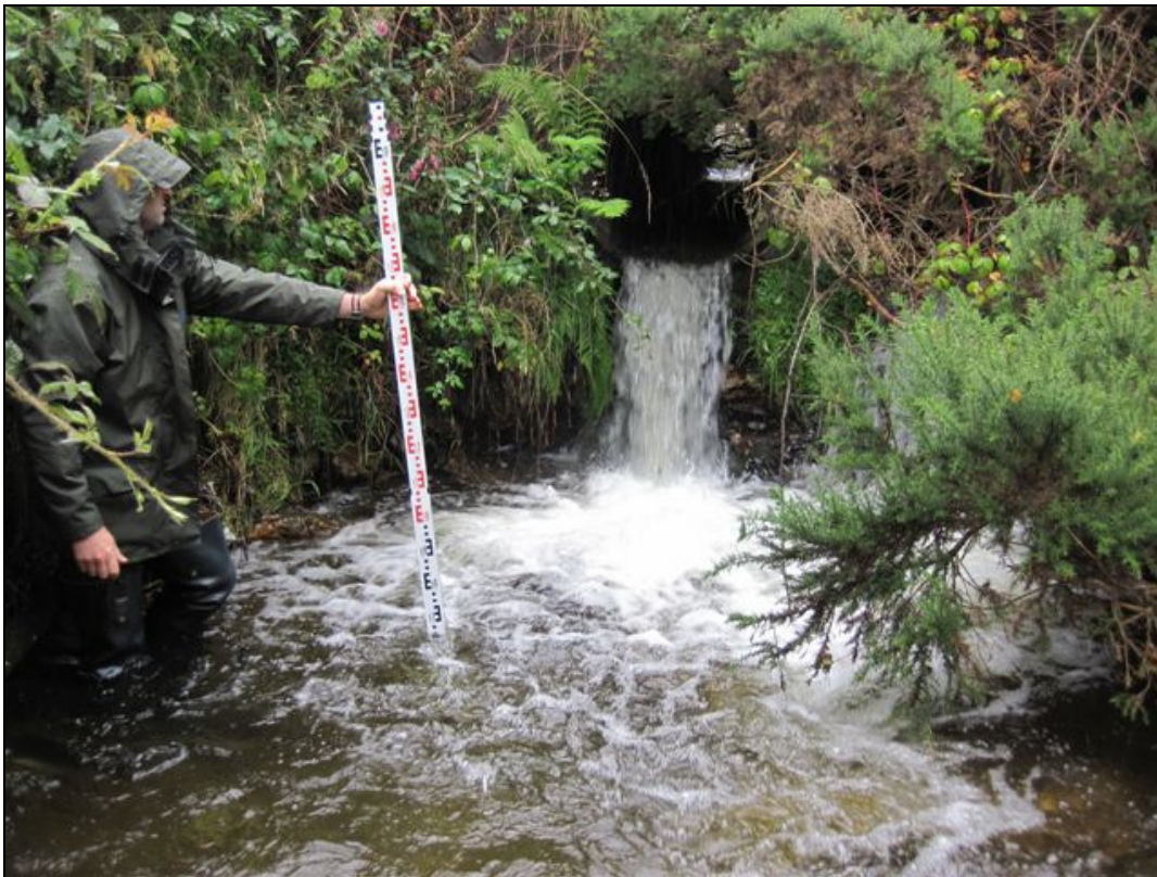
Figure 18. Perched pipe culvert at Greens Bridge, headwaters of the Ballycreen/Macreddin Brook. Significant fall/jump downstream of pipe. Bank erosion noted downstream also.
