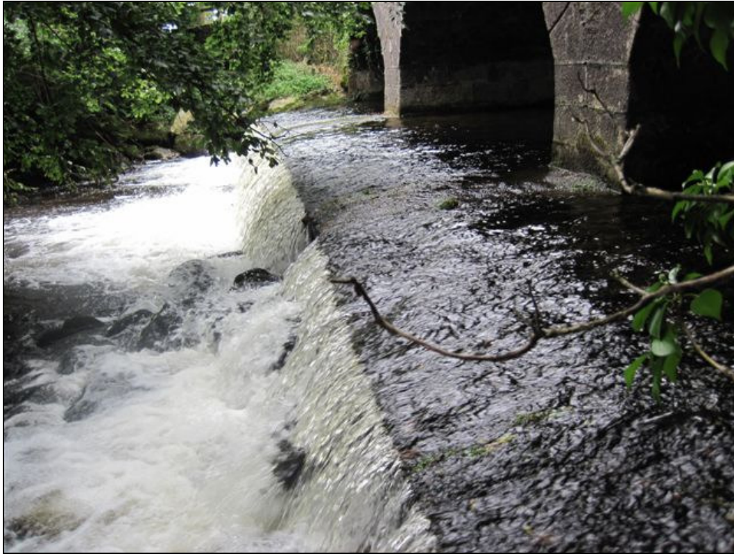
Figure 9. Ballinglen Bridge: This photo demonstrates the fish passage issues associated with laminar flow, flow velocity and the perching associated with this scour protection apron.
