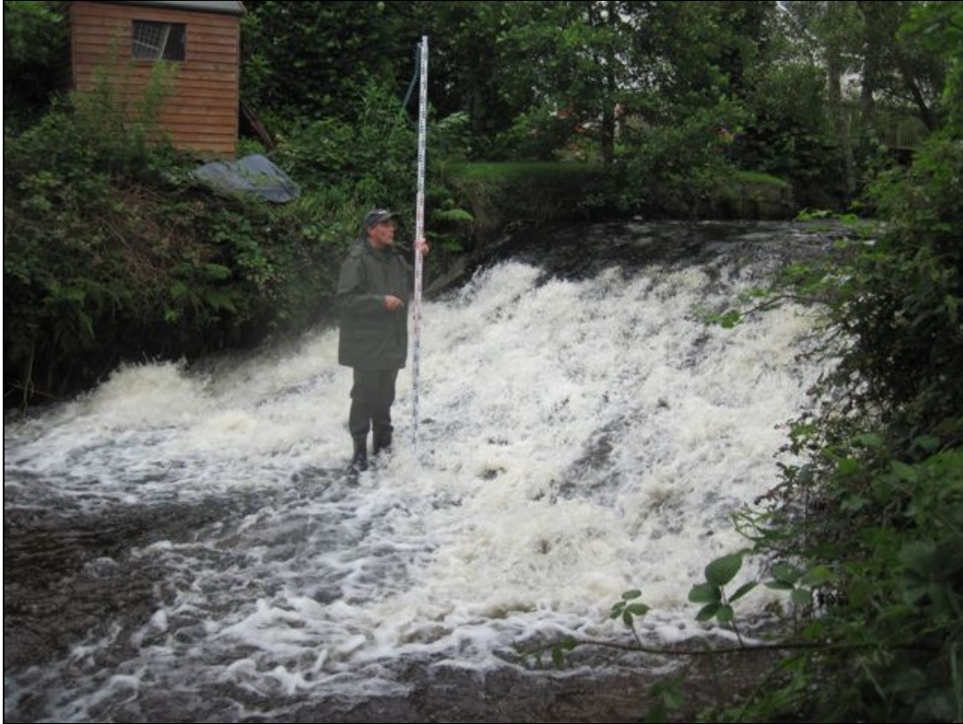
Figure 27. Dam across the Macreddin/Ballycreen Brook in Aughrim. This structure represents an impassable barrier to fish passage. Excellent salmon spawning/nursery habitat upstream of this site. Catchment wide electrofishing survey of the Avoca system in 2002 highlighted the absence of juvenile salmon on the Macreddin/Ballycreen Brook upstream of this structure.
