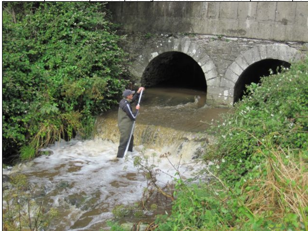
Figure 10. Threemilewater N11: photo demonstrates the combination of high velocities on a moderately sloped apron, laminar flow and perching, creating an impassable barrier to fish. This site would benefit from a mammal pass on this very busy/fast stretch of road
