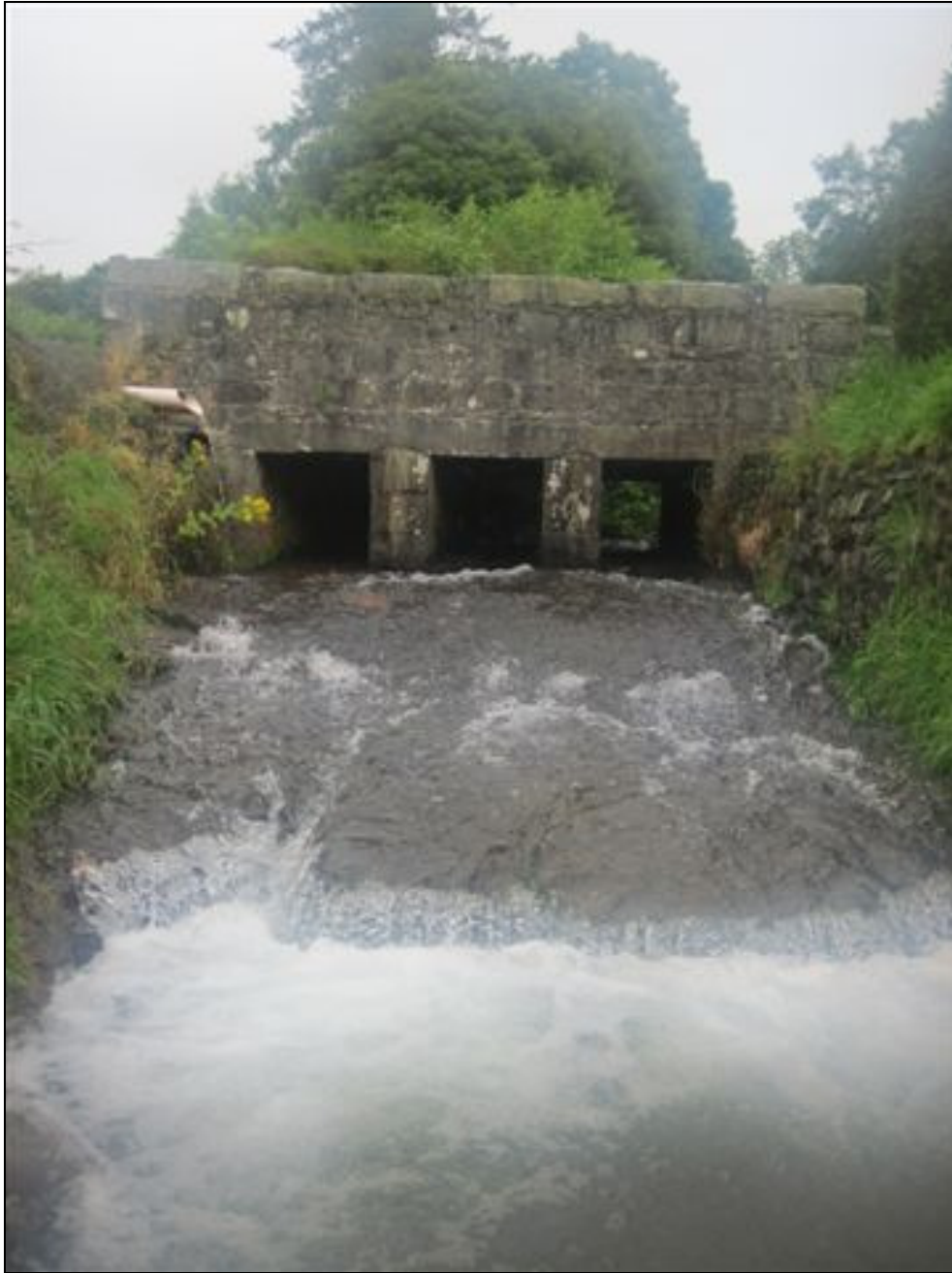
Figure 12. Old masonry bridge structure near Avoca: composed of three masonry 'box' culverts with a long and moderately sloped concrete scour protection apron downstream. This photo shows the high velocities and laminar flow associated with this structure.
