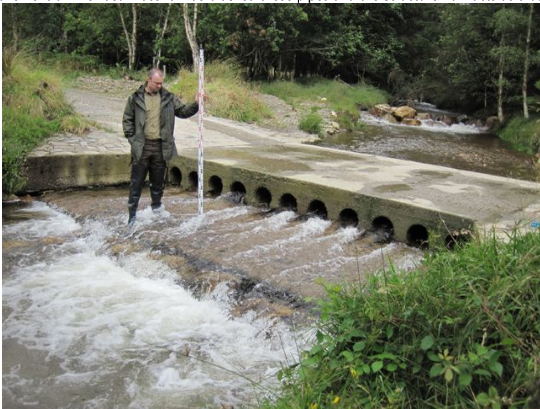
Figure 22. Ford structure on Avonbeg tributary, utilising undersized pipes encased in concrete, with scour apron downstream. Many of the culvert pipes were fully or partially blocked. Structure represents a significant impediment to the free passage of fish.
