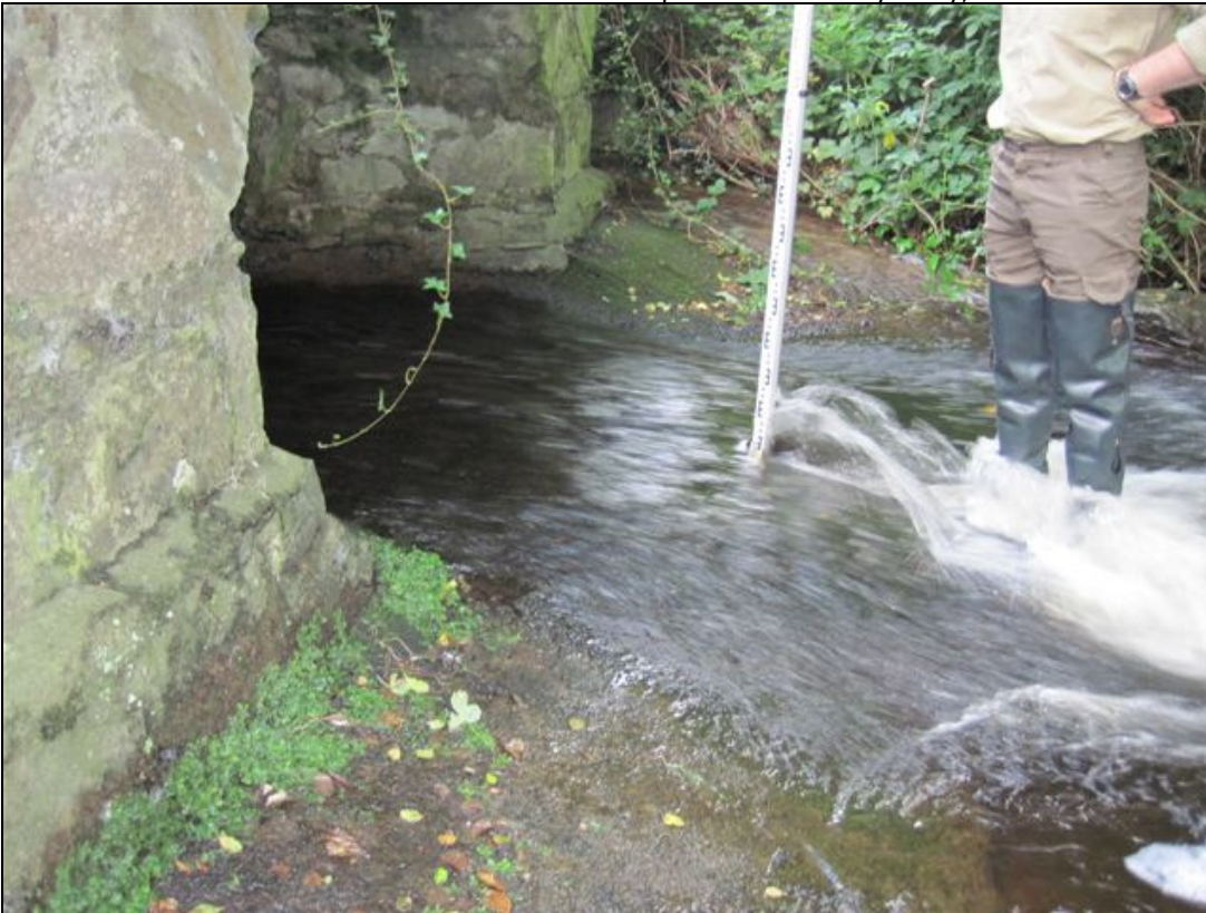
Figure 14. Leabeg Stream at Leabeg Bridge: please note flow velocity and laminar flow associated with this moderately sloped concrete scour protection apron.
