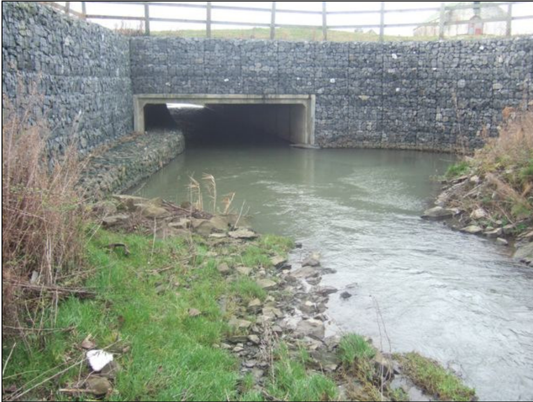
Figure 26. Griffen River, Liffey trib. Co. Dublin. Backwatered box culvert. Culvert bed 500mm below river bed level. Natural bed material deposition within structure, fish habitat and passage over length of structure maintained. Structure includes a mammal pass, the incorporation of which would have been very difficult within a round/elliptical culvert
