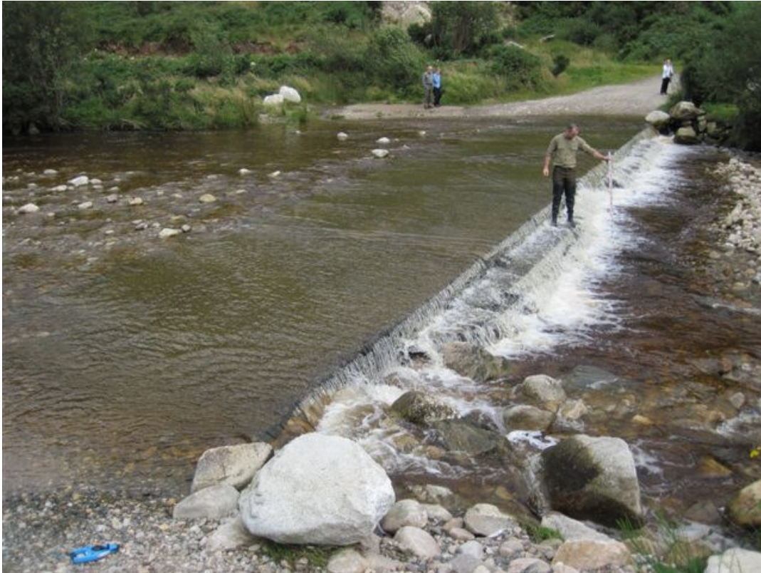
Figure 21. Ford on Avonbeg Main Channel at Glenmalure. Structure is composed of a series of undersized concrete pipes lain parallel to each other and encased in concrete. The downstream movement of river bed material has blocked these pipes and the structure now acts as a dam.
