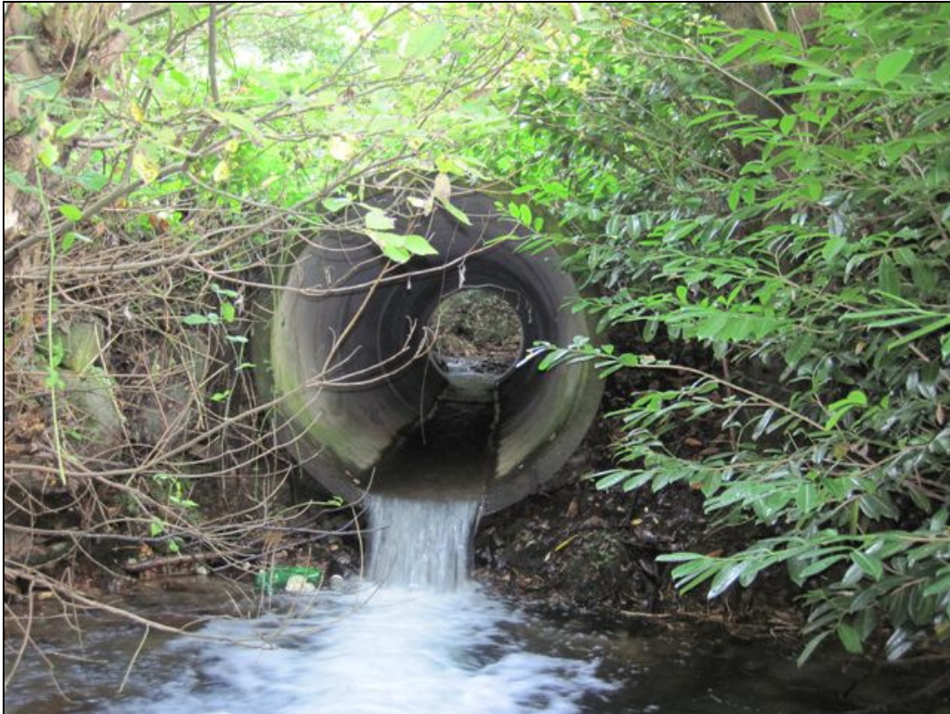
Figure 19. Large perched concrete pipe culvert crossing of Avoca trib. on private road near Avoca. Sea trout noted in pool downstream of culvert. Fish passage difficulties at this site could have been avoided had this culvert been lain below bed level and backwatered.
