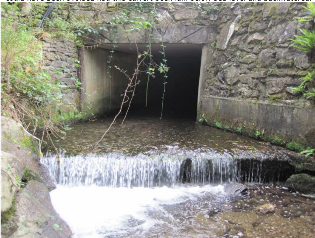
Figure 20. Box culvert with perched concrete scour protection apron. Private roadway on a Goldmine River trib. Structure represents significant impediment to fish passage.
