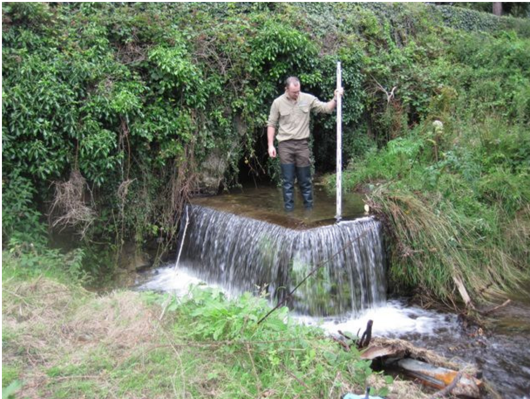
Figure 29. Structure at Preban Bridge (Derry Water system) near Ballinglen purpose of which we were informed was to provide for a gravity feed water supply to nearby farm
