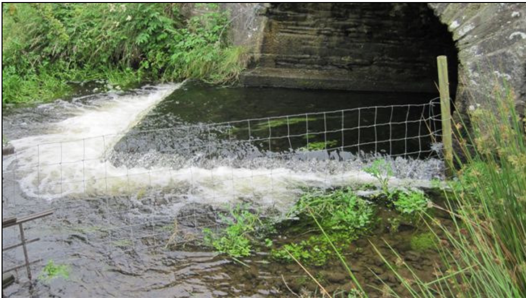
Figure 15. Mullyclagh Bridge: site in headwaters of the Slaney catchment before the installation of a series of low level weirs downstream of the perched scour protection apron. Electro-fishing of this site found excellent populations of trout, and salmon parr, downstream of this apron.
