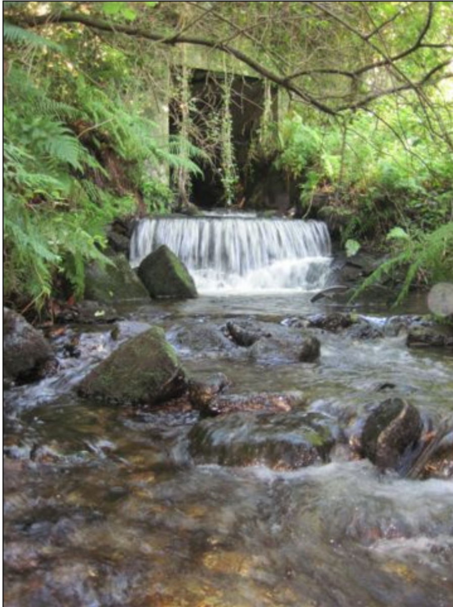
Figure 11. Photo showing a perched concrete scour protection apron on a tributary of the Avonmore River. The watercourse at this location represents excellent salmon nursery habitat. The main Annamoe to Laragh road is located immediately downstream of this site and the Armco Style culvert used for that crossing also represents an impassable barrier to fish passage.
