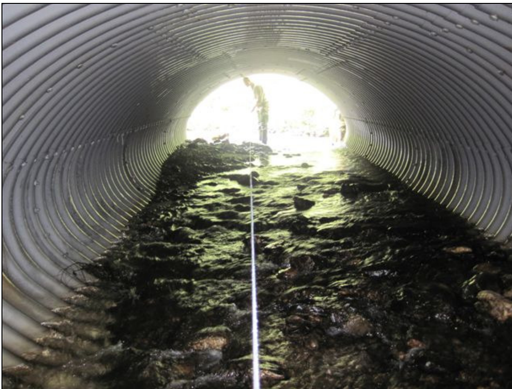
Figure 25. Furnace Bridge, Armco style culvert, which replaced an old masonry bridge, structure constructed well below bed level, backwatered throughout, natural bed material deposition within structure, fish habitat over length of structure maintained. Free passage of fish guaranteed. This site would also benefit from a mammal pass on this very busy/fast stretch of road.
