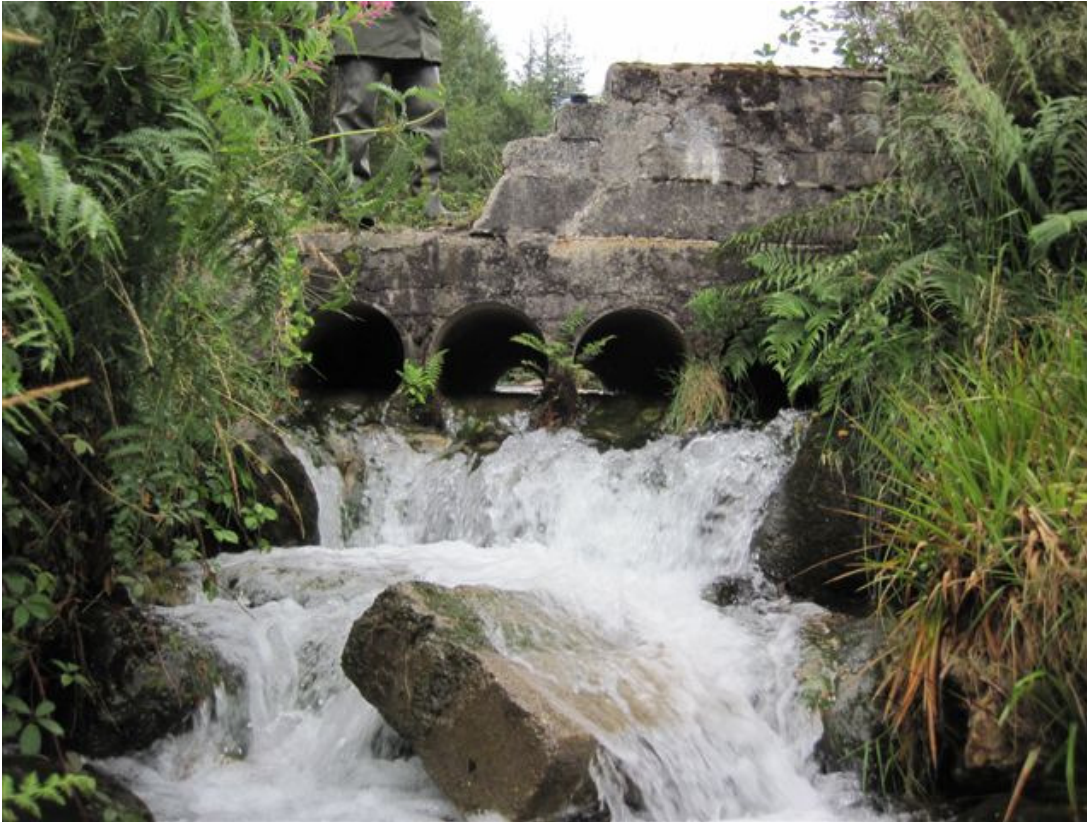
Figure 23. Perched pipe culvert crossing with scour protection apron over Mucklagh Brook, Ow river tributary. Structure represents barrier to the free passage of fish.
