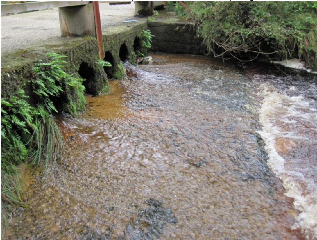
Figure 24. Ford Structure on Avonbeg trib. utilising undersized pipes encased in concrete, with scour apron. Majority of the culvert pipes fully or partially blocked. Structure represents a barrier to the fish passage, with excellent salmon spawning/nursery habitat u/s and d/s. Pipe size too small to facilitate most fish passage.
