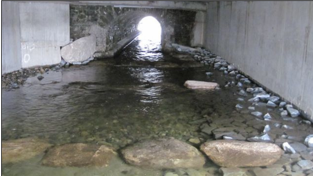
Figure 16. Mullyclagh Bridge after road/bridge widening and incorporation of low level weirs.
